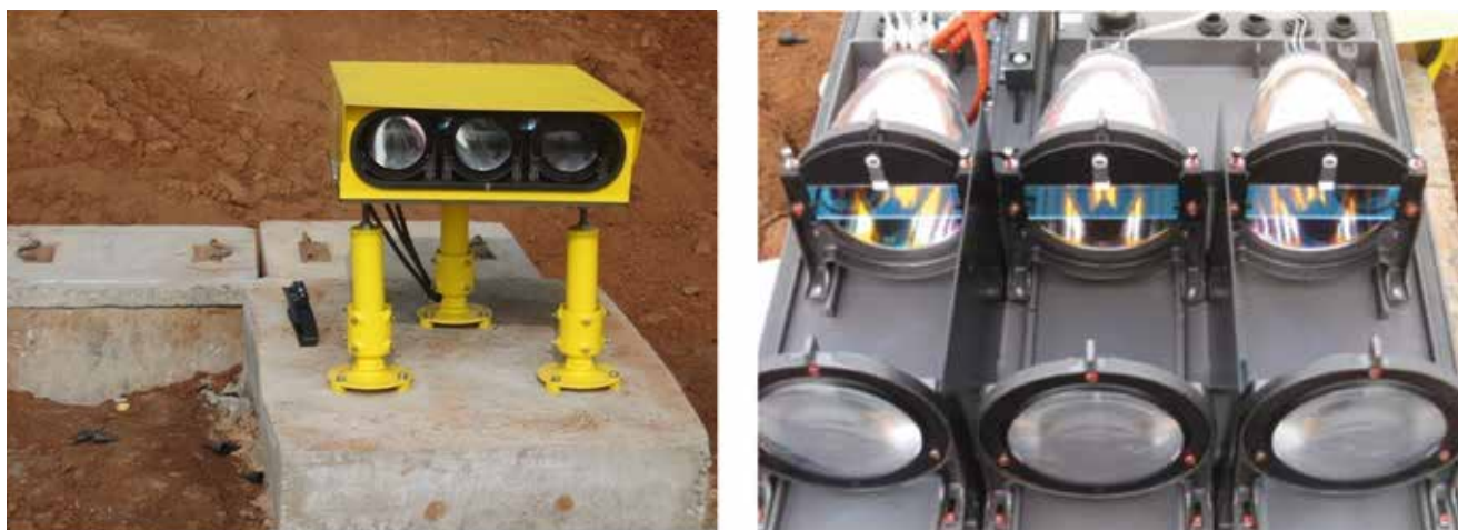
Figure: 6 Installation and Components of PAPI Light
